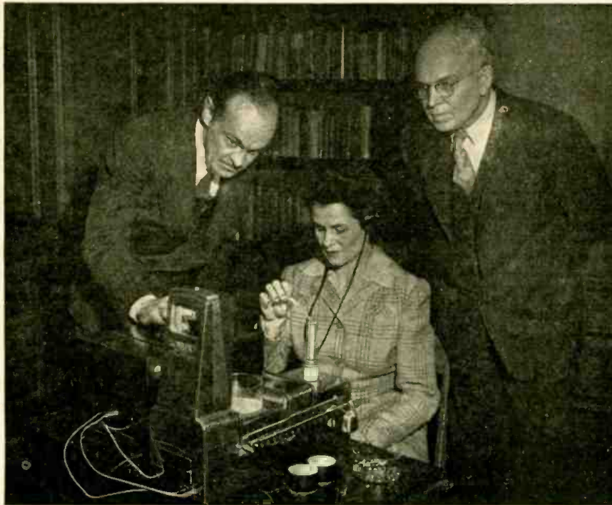
The photo shows (center) Mrs. Jane Muhlfeld Barbour, who has been blind from birth, seated before the new "Audio" scale in much the same manner that a blind operator would in an industrial plant. On the left is J. O. Kleber, Chief Engineer of The American Foundation For the Blind; and (right) Lawrence Williams, Chief Engineer of the Toledo Scale Company, who developed this new device.
